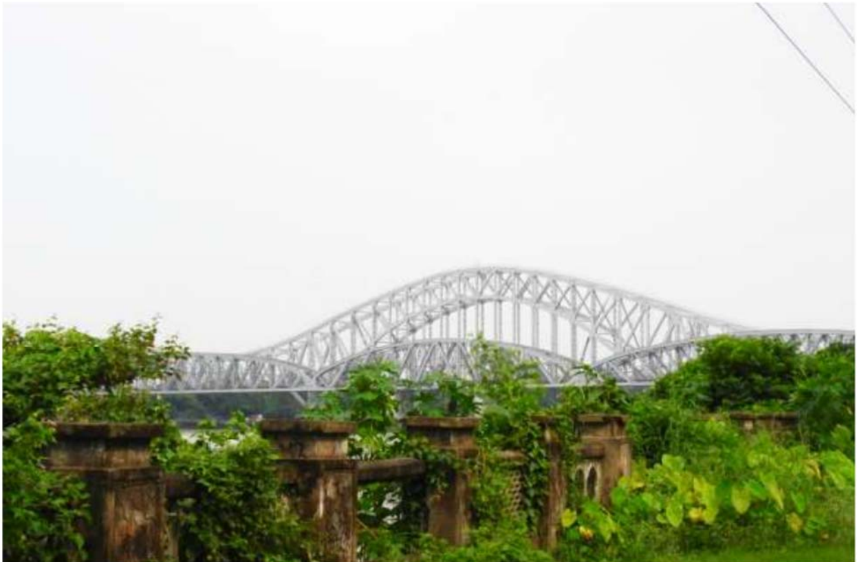
Plate 27 – Sampreeti Bridge on River Hugli.
