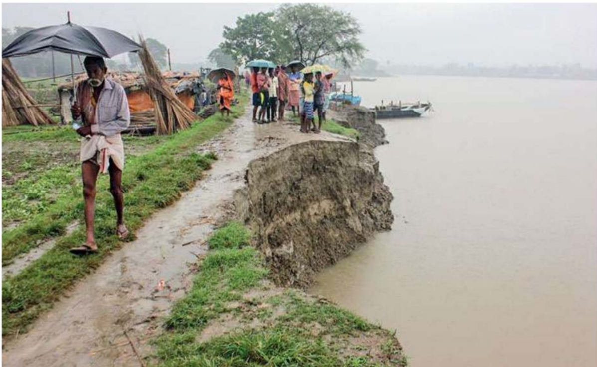
Plate 58: Bank Erosion along Hugli River , Balagarh during Monsoons , Source : Anandabazar .
